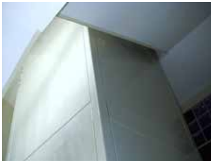
Ill. 4a: Lift shaft with closed sheet steel panels ...
