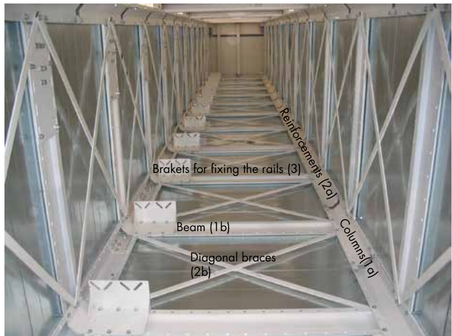
Ill. 2: Components of the DICTATOR lift shaft system
