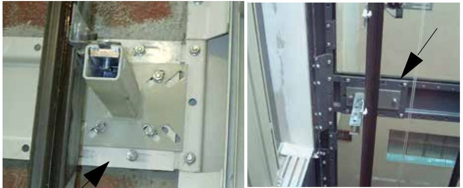
Ill. 3 a/b: Examples of fixing brackets/plates for the rail fixtures of the lift companies
