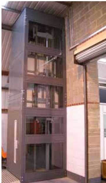
Ill. 4c: Lift shaft with window panes
