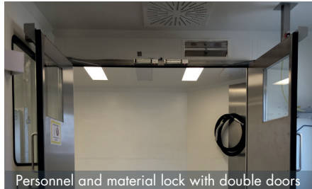
Personnel and material lock with double doors
