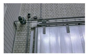
The very large sliding fire doors in an explosion-proof warehouse were equipped with DICTATOR door operators. These not only had to meet high ATEX standards, but also comply with fire safety regulations.
