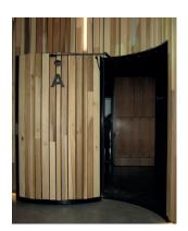
These fire doors integrated into the wood-panelled wall of a theater in the Netherlands required a customized automation solution, as it was not allowed to install anything on the outside of the doors because, for architectural reasons, it should not be recognizable that these are doors. In addition, some of the doors were integrated into a round wall surface, which meant that they were also curved. Therefore, neither a standard door closer nor a standard door operator could be installed here.
