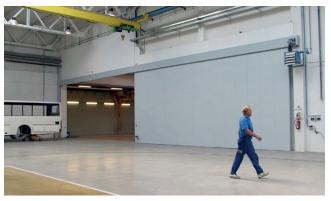
Special solutions for fire doors and gates are no problem for DICTATOR. Because of the huge door width of 11.5 m, a "normal" fireproof operator with mechanical closing device was not feasible here. Instead, it was necessary to use a special operator with a control system that would always ensure the safe closing of the fire door, even in the event of power failure.
