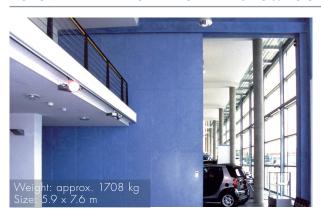
This very large gate also had to meet special requirements. On the one hand, a pedestrian door had to be built into it. On the other, there is a gap in the wrap-around balcony into which the gate enters when opened. With the gate closed, a ramp needs to fold out to bridge the gap, and when the gate is open, this ramp needs to retract again.
