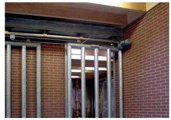
This application on a rhino enclosure was somewhat unusual. 0.18 kW motors were used and a sturdy chain was selected for power transmission, because the gates also have to stand the strength of the rhinos sometimes. Additional chain guides were installed to prevent the chain from becoming slack.
