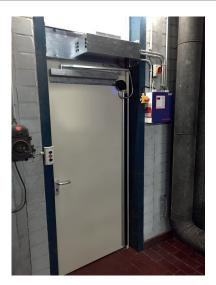
Due to the high negative pressure in the power plant building, the doors could barely be held open (which could be quite dangerous) and the overhead door closer had no chance of closing the doors properly under unfavorable conditions.
