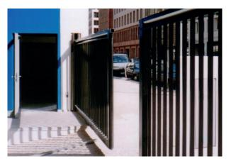
Unlike normal gates, this entrance gate is opened mechanically by a spring rope pulley, while the operator closes it. The closing motion is time-delayed by an additional time relay, since the cladding in the wall has to be opened first.
