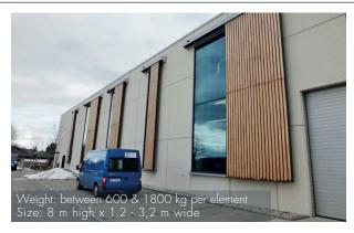
DICTATOR door and gate operators are not only used for "conventional" doors. They can also be used to automate other kind of elements, as in the case of these sliding sun shades. The particular difficulty of this application was the size of the shading elements, which were installed on the exterior of the façade.
