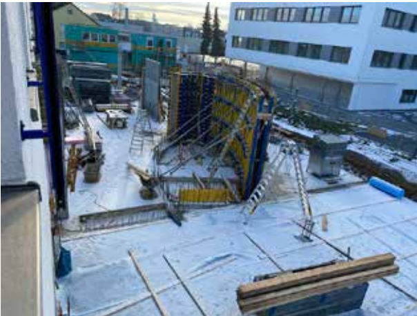
The construction site is covered with some snow.
