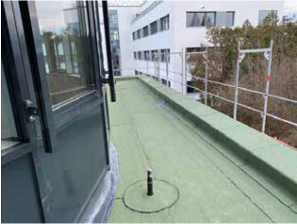
And now everything is ready for the green roof.
