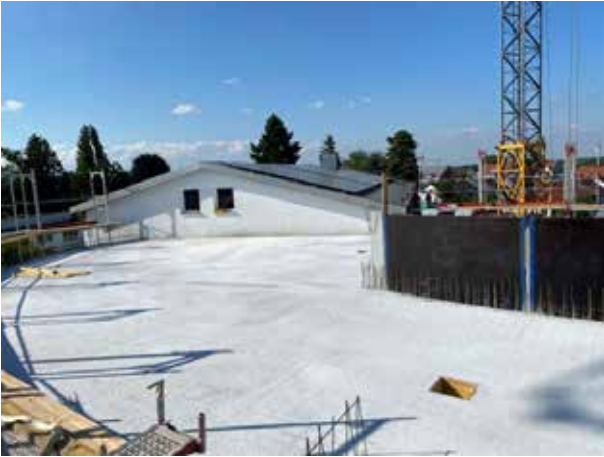
The ceiling on the second floor is finished.
