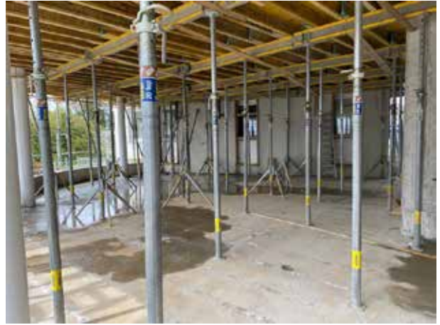
In the future sales office under the tons of structural steel and concrete, everything is fine.
