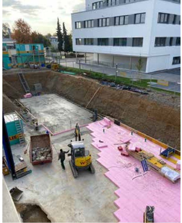
And the base plate is finished.
