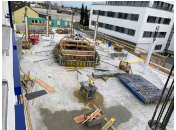
The "bridge" over the stairway is finished.
