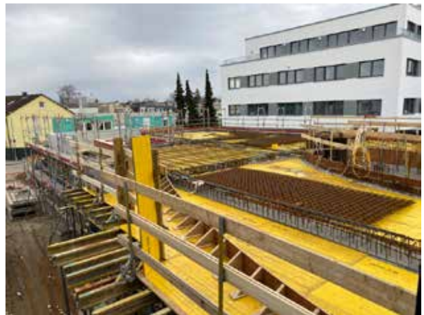
Here you can already see the ellipse that determines the shape of the first and second floors.
