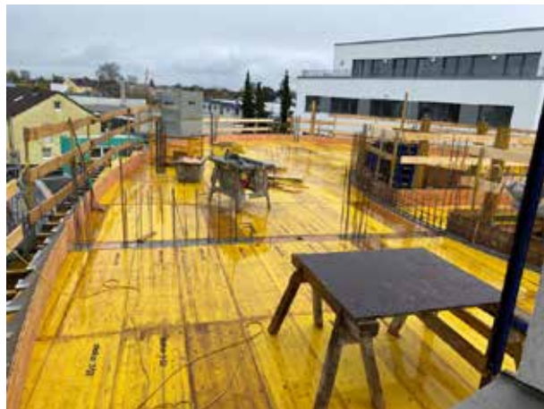
... until it is completely assembled all around.
