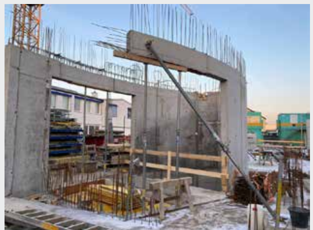
The staircase ellipse from the other side.
