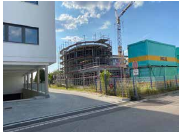
The shell is now complete in full height.
