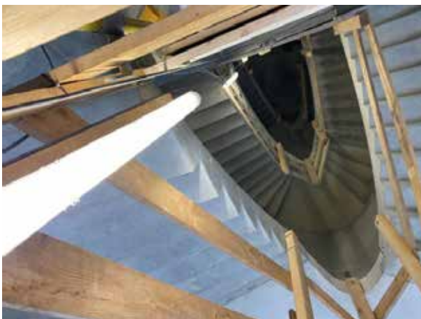
View from the top of the staircase.
