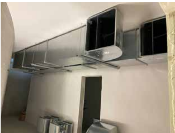
The first ventilation ducts are installed in the basement.
