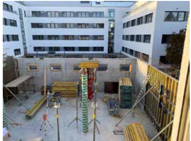
Covering the ceiling of the ground floor has started.
