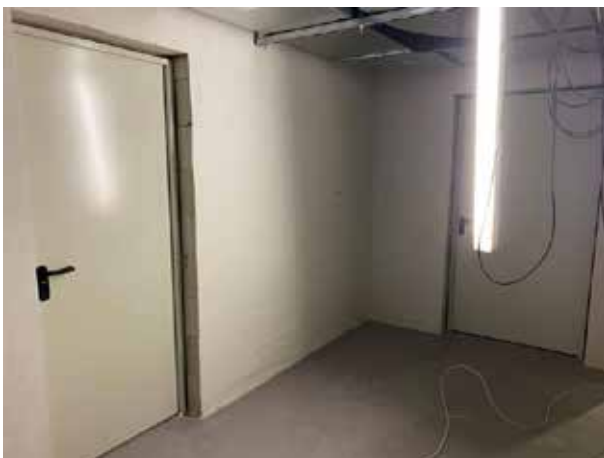
The doors have already been installed in the cellar.
