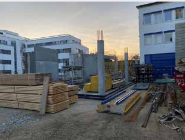
View from the outside of the future entrance. On the right in the picture our previous building, which will be completely renovated after completion of the extension.
