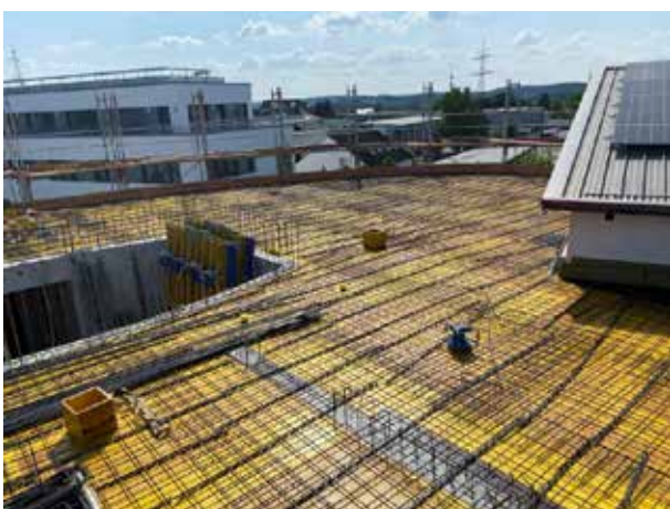
Above the stairwell ellipse nothing is boarded – because there the roof is glazed, so that always a lot of natural light enters the stairwell.
