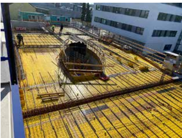
The first of many layers of structural steel are laid.
