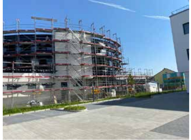
... and from the neighboring property behind
