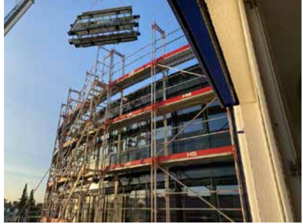
The frames for the glass roof above the stairwell float in.
