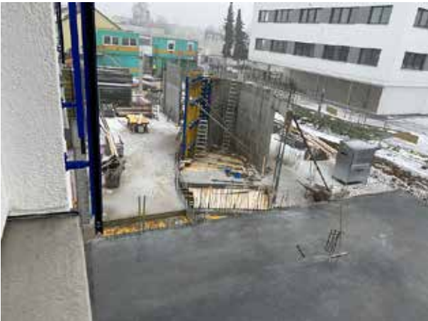
The floor in the future storage area has been cleared of snow, the formwork on the ellipse of the staircase has been removed, and work has begun on the formwork on the other side.
