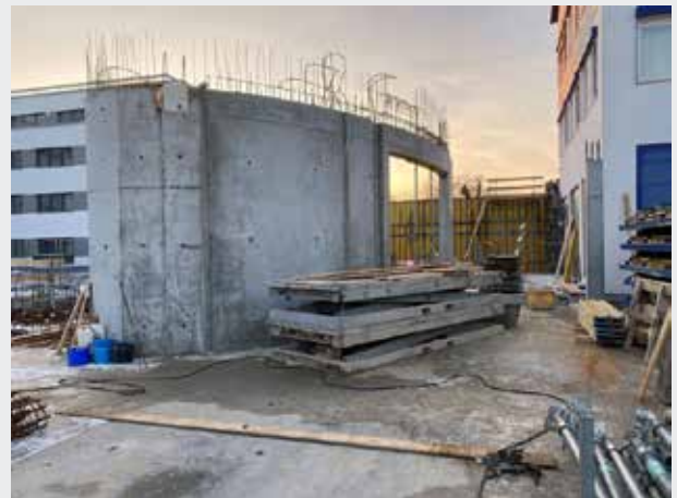
Here we are in the future entrance and exhibition area.
