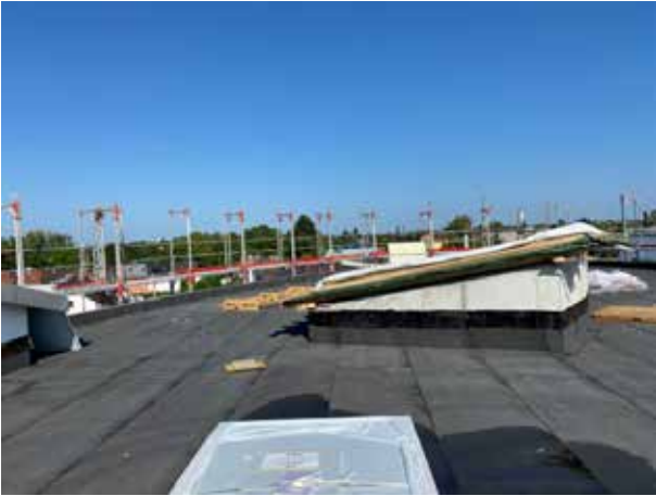
The stairwell is still covered by foils. Later, the light will enter the stairwell through a large glass cover.
