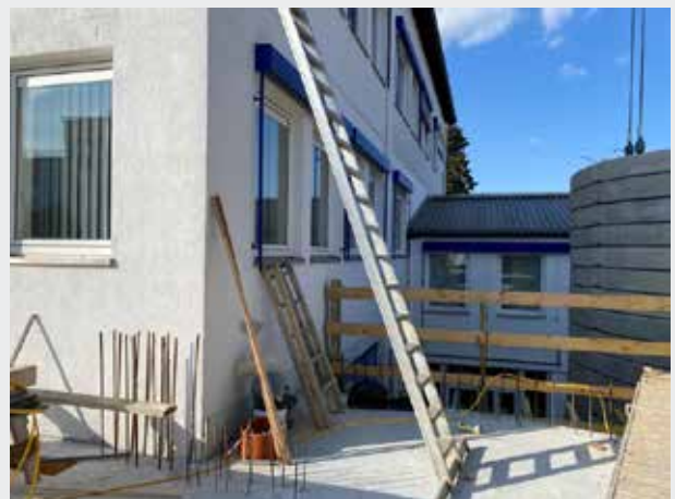
The ellipse encloses part of the existing building.
