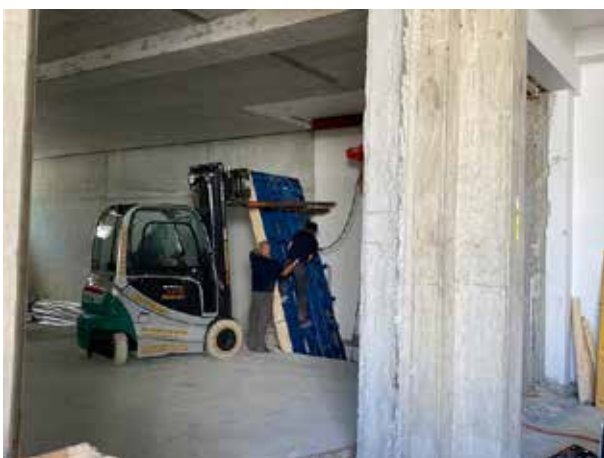
Inserting the side panels is precision work.
