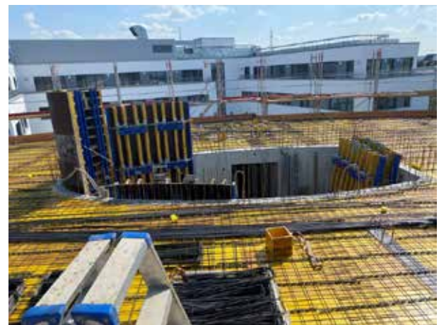
Here once again clearly visible: the upward "open" staircase.
