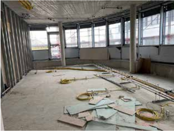
The future staff lounge, with its own roof terrace.
