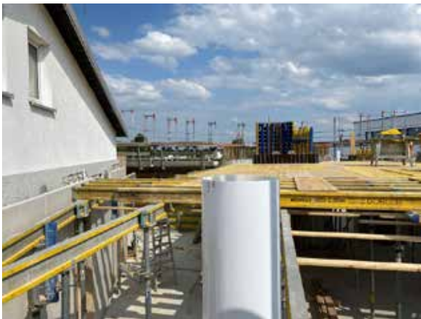
Here, the new building "docks" with the existing building.
