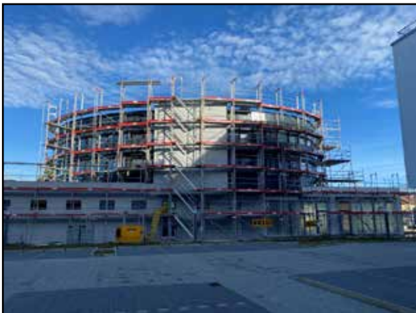
A view of the annex from the neighboring property. I wonder what it will look like when the scaffolding is taken down after the winter break?
