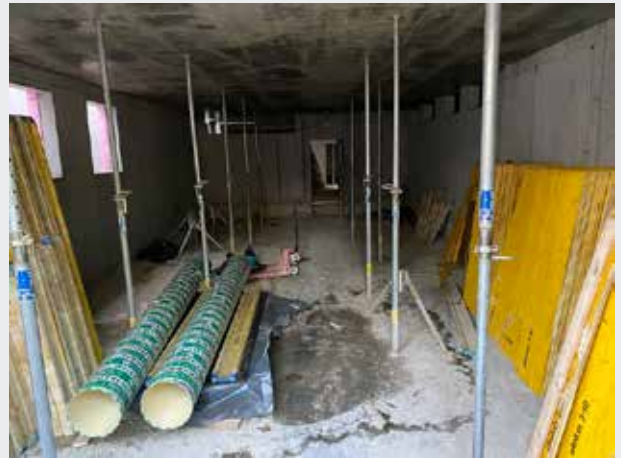
A view of the front basement area. This is where the ventilation system will find its home.
