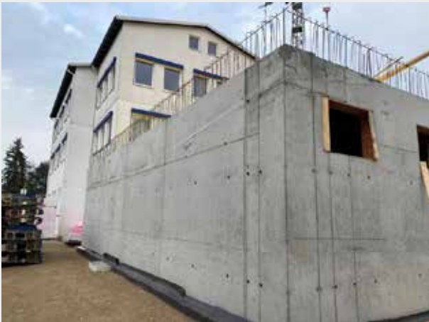
And finally, once again the view from the back of the first floor walls of the extension and behind it the existing building.
