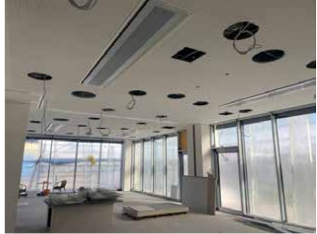
A little later, the final sound-absorbing ceiling is installed.
