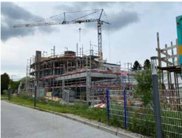
This is how our construction looks from the neighboring property.
