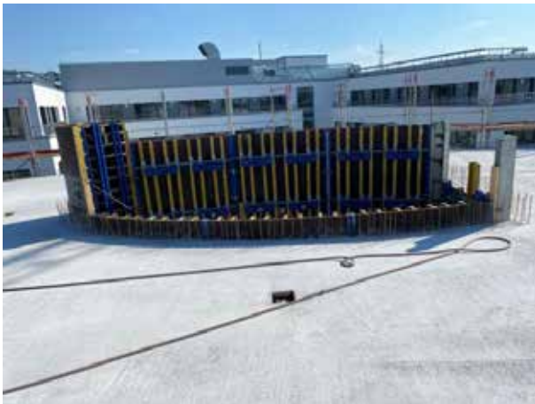
The supports for the sloping glass roof still need to be concreted.
