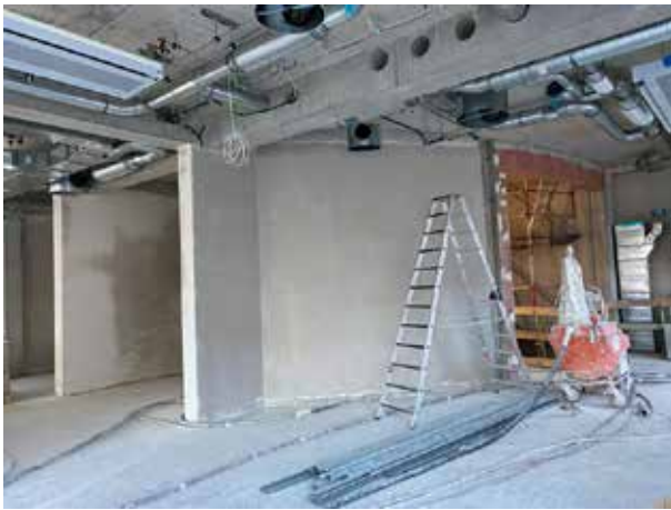
Now the walls on the first floor are also being plastered.
