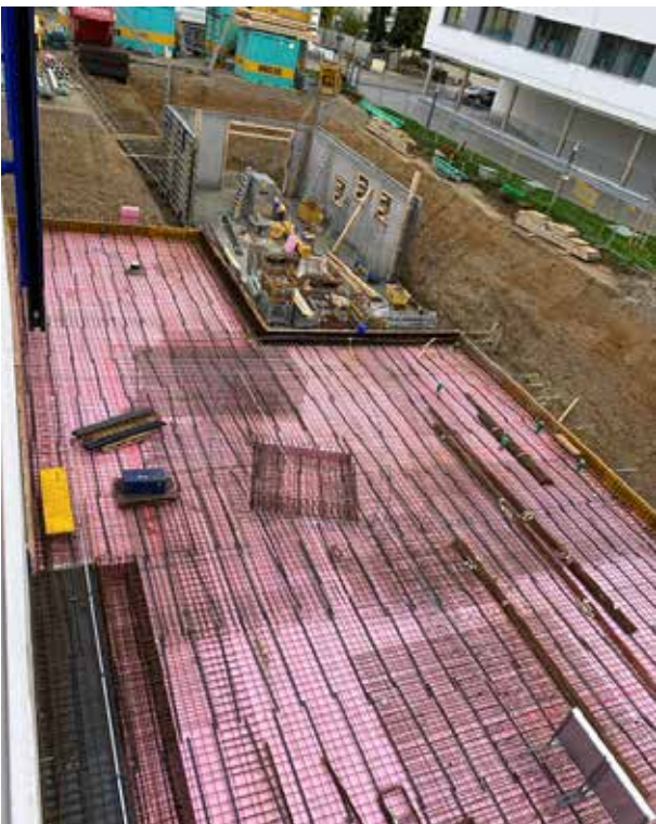
The first basement walls are in place.
