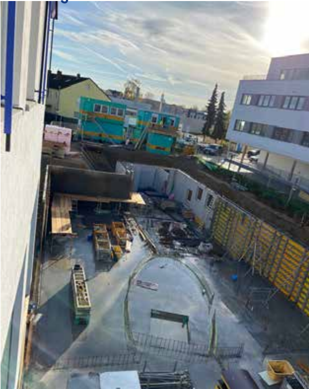
The remaining exterior walls are being shaped and poured.
