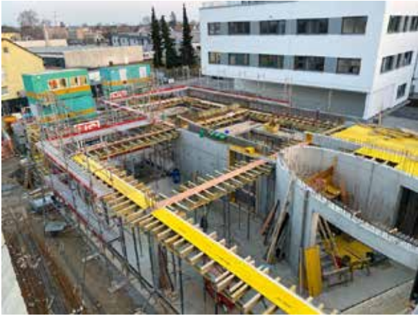
The beams of the slab in the front area are formed.
