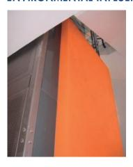
The necessary ventilation of every lift shaft is achieved by using perforated sheet metal panels below the upper beams. The size of these panels depends on the base area and the travel of the lift.
